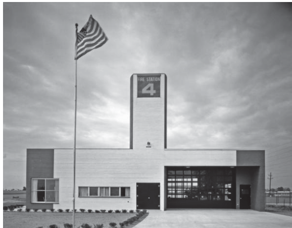
Figure 2. Firestation No. 4, Courtesy Venturi Brown & Associates Inc.
